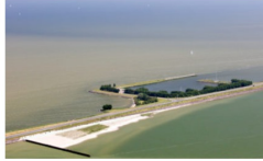
Houtrib Dike Pilot Project
